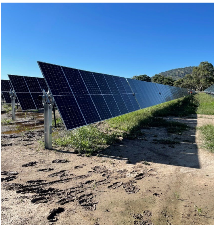
Figure 20 – Example of a typical single axis tracker system with PV modules mounted in single panel portrait orientation (1P configuration)
